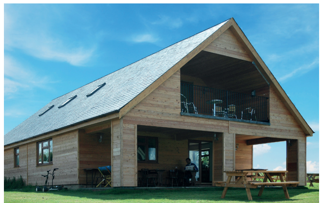
Halflap cladding fitted with expansion gaps Grade B Siberian larch halflap
