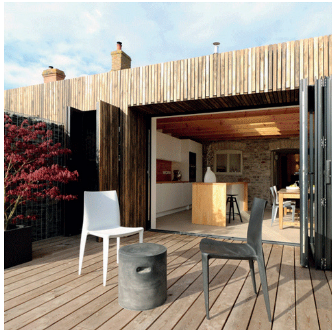
Halflap profile, face fix Siberian larch cladding
