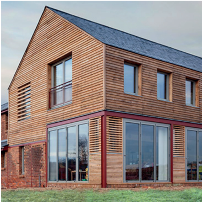
Feather-edge profile with plenty of overlap British larch cladding
