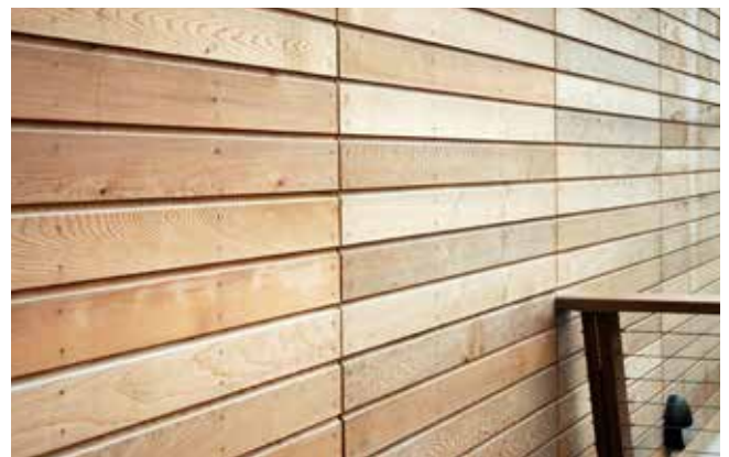
Modern: Dried wood with a smooth machined finish Canadian cedar halflap cladding
