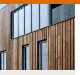
The Brimstone® range is produced by thermally modifying fast-growing British hardwoods to produce durable, stable and consistent timber products that are ideally suited to exterior cladding applications. The Brimstone range includes ash, poplar and sycamore.
